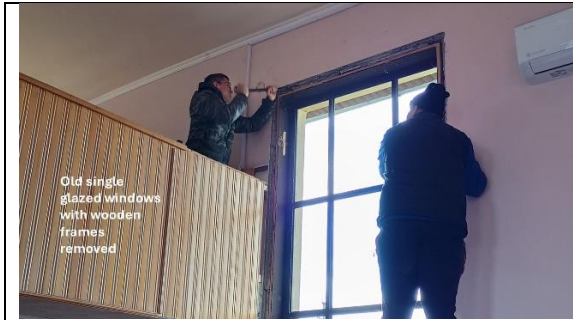
Windows out but now bricking to right size the space for new windows
