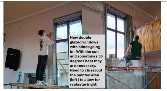
Thirteen windows being removed and two doors, but note the wood surround and raised plinth that will all have to be removed
